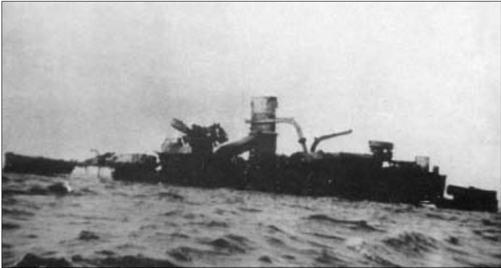
Photo 1. Schleswig-Holstein in 1961, the fore and aft gun towers can be seen, as well as the remains of a funnel.
